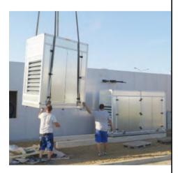
The specially provided crane lugs are to be used to transport the acoustic housing. These may not be mounted on the upper corner connections.
