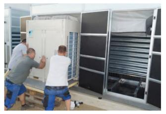
Align refrigeration, air conditioning or heat pumps in the middle of the air separation part
