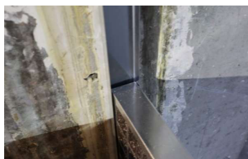
detail 2: U-profile on the side walls between the walls of the transmission room and panels
