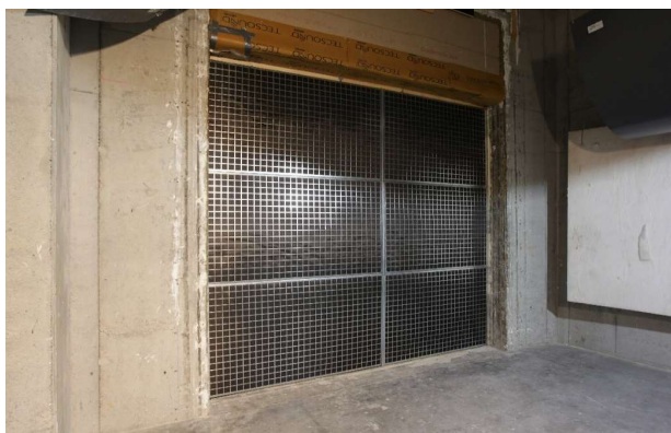
front side in the transmission room
