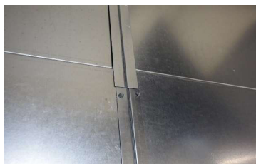
detail 1: I-profile at the location of the vertical joint between the 2 columns of noise barriers
