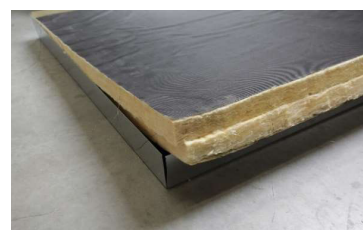
detail 3: different layers of the noise barrier 100mm non-combustible glass fibre insulation with resistant and water-repellent coating
