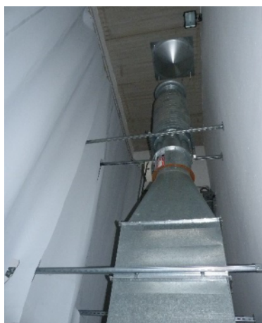
Photo 3 : Convergent, fan & silencers (4 - 8)
