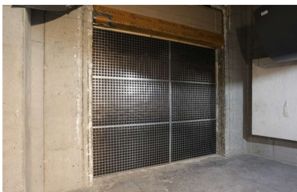
front side in the transmission room
