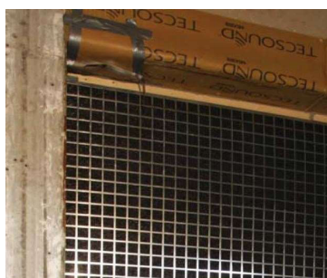
detail 4: detail on the top of the noise barrier. The opening was filled with a wooden beam and sealed with flexibel mastic tixotrophe
